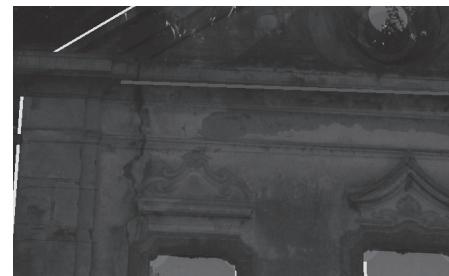
Figure 11: The match for the same camera position and orientation shown in Figure 10. The structural edges of the model are shown over the picture.
